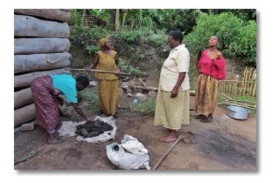
3) Mix the fibres into the pile of clay. Beat the clay / fibre mix again with a hoe to make sure all the fibres are mixed in thoroughly.
