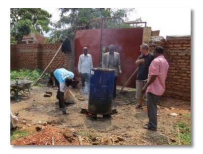
7) As the fire under the drum burns, smoke will come from the opening in the top of the drum.
