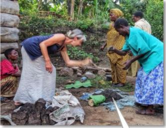
6) Lay one half of the pole onto a piece of sacking or a strong sheet so that the clay does not stick to the ground. The pole should be wrapped in a banana leaf (or plastic bag) so that the pole can easily be removed once the moulding has been completed.
