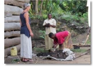
4) Collect a banana pole (or plastic drainage pipe, etc) to act as a mould for the clay.
