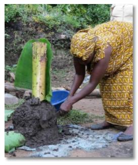
9) Once a large pile of well-compressed clay / mud has been created, start to shape the mud pile into a cube with a large knife.
