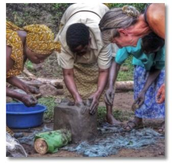
13) Continue to smooth the internal and external surfaces of the fire to make a good finish.
